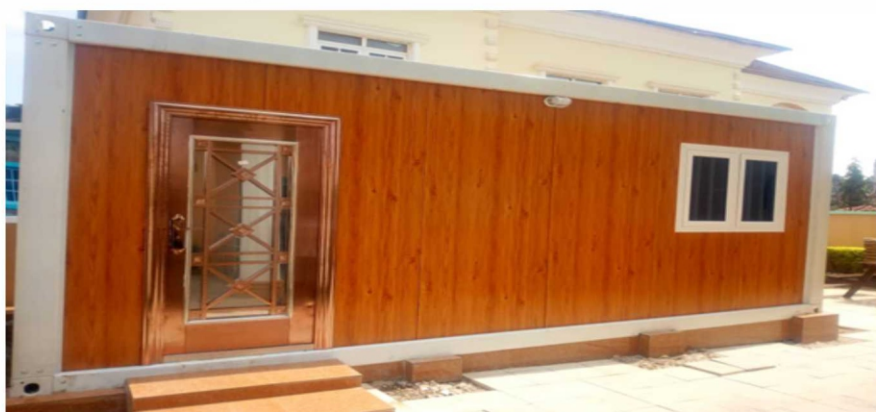
External view of an office space in Abuja using Polyurethane sandwich panel with MDF Printek steel
